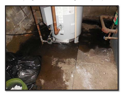
Leaking pressure release valve (Community Gateway Motel, Saratoga, Saratoga County DSS)
