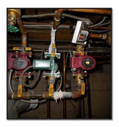
Corrosive build-up on boiler pipes (Budget Inn, Malta, Saratoga County DSS)
