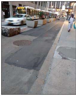
**Figure 4.** Photo of tan granular paint missing from pedestrian plaza.
