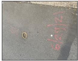
**Figure 3.** Permanent gas cut still missing a gas valve cover after almost a year.
