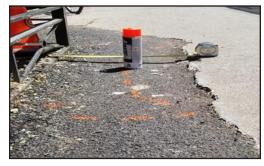
**Figure 5.** 1–2" depression causing a trip hazard on the sidewalk.
