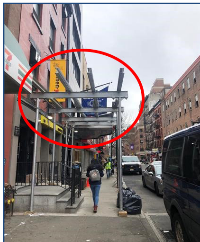
Figure 3 ( top left ): Shed with an uncovered bolt. Figure 4 ( top right ): Shed with an unattached rail. Figure 5 ( bottom left ): Shed with a hole in the ceiling. Figure 6 ( bottom right ): Shed without ceiling
