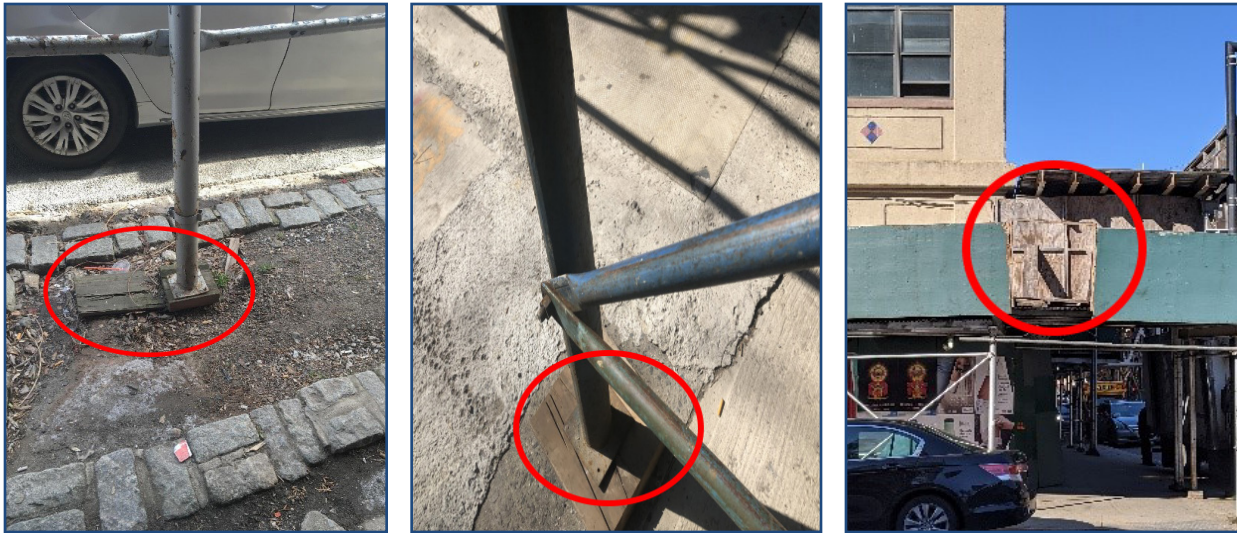
Figure 7 (left): Shed with broken/disconnected base. Figure 8 (middle): Shed with missing screws/nails to connect pole to the base. Figure 9 (right): Shed with missing parapet section
