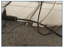
Figure 1: Loaded power strip plugged (or "daisy-chained") into another loaded power strip.
