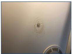
Figure 2: Water damage/possible mold.
