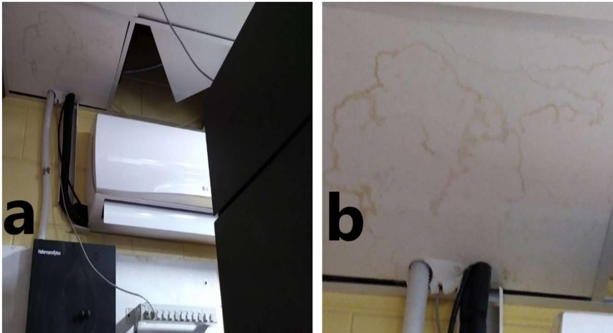
**a) Water damaged ceiling above server equipment
